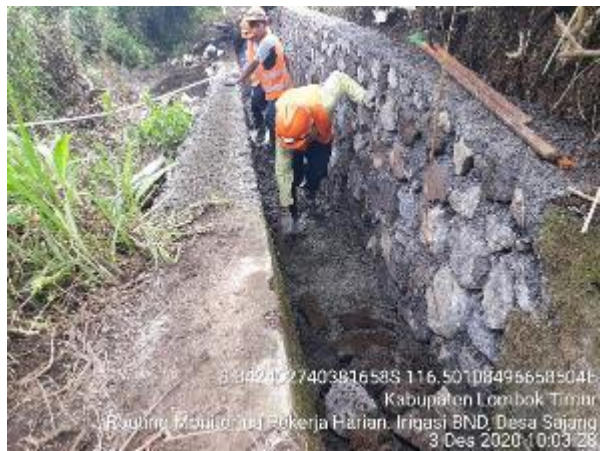
4 Construction work progress 50%
