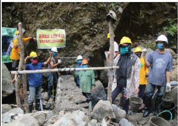
3 Construction work of catchment reservoir
