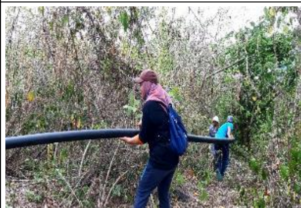
5 Clean water piping installation
