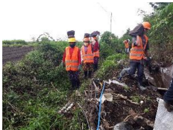
2 Preparation work i.e. material mobilization
