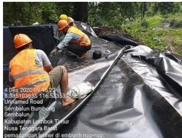
4 Reconstruction work progress 50%
