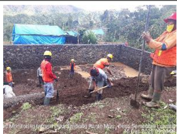
4 Construction work progress 50%
