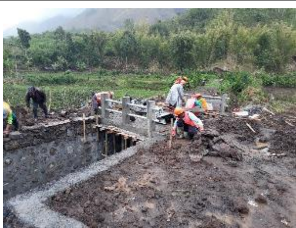
4 Construction work progress 50%
