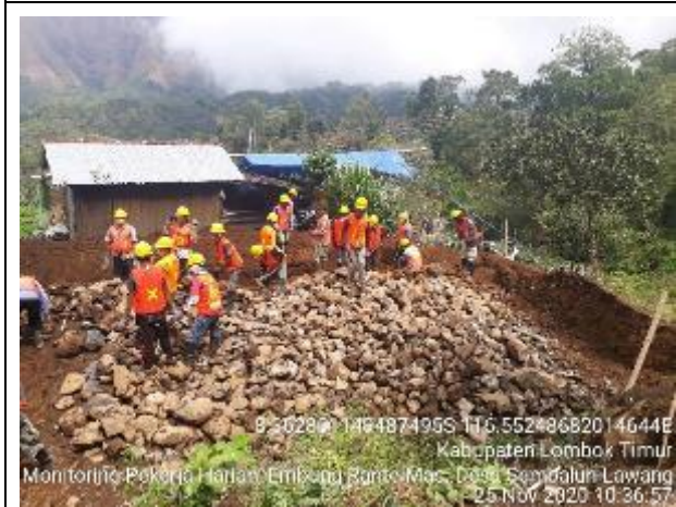
3 Construction work progress 5%
