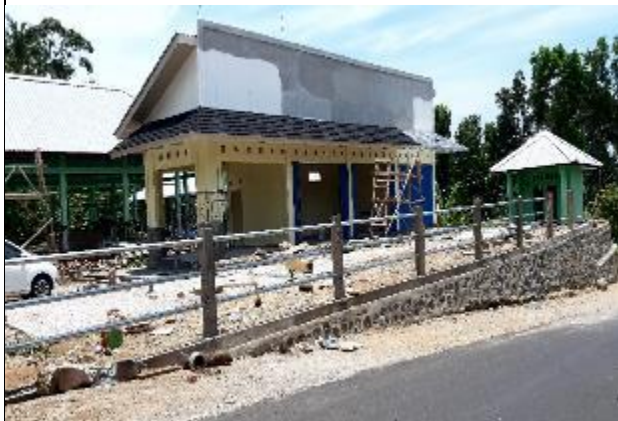
5 Construction work progress 75%
