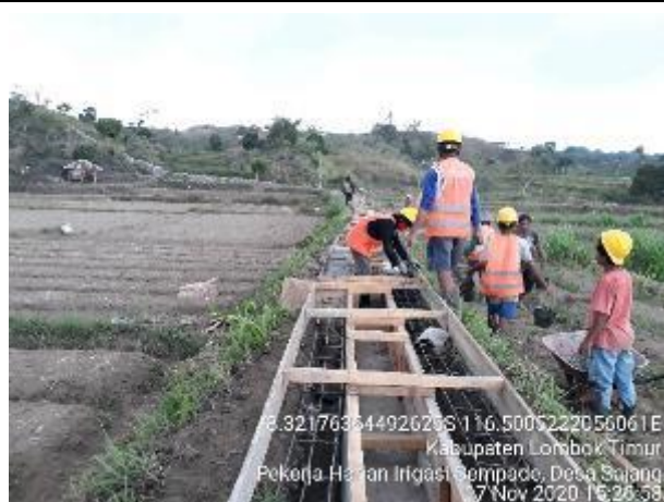
4 Construction work progress 50%
