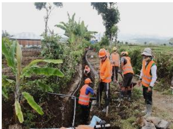
3 Construction work progress 25%
