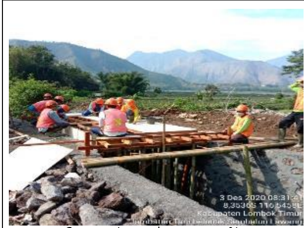
3 Construction work progress 25%
