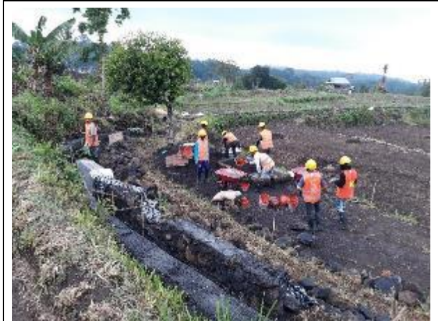
3 Construction work progress 25%
